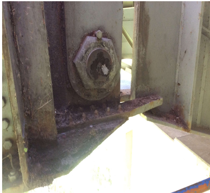
PHOTO 5 Description Joint 20a Girder 3 active corrosion, nuts reduced to nodes.
