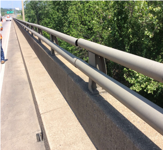
PHOTO 1 Description Span 20 Northbound loose bridge rail connections.
