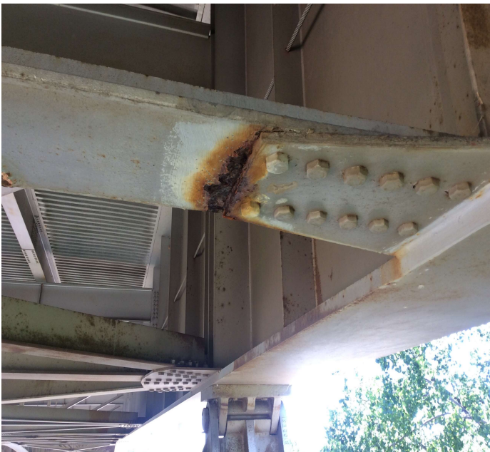
PHOTO 7 Description Span 17 Girder 1 joint 17A active corrosion with section loss to stringer connection.
