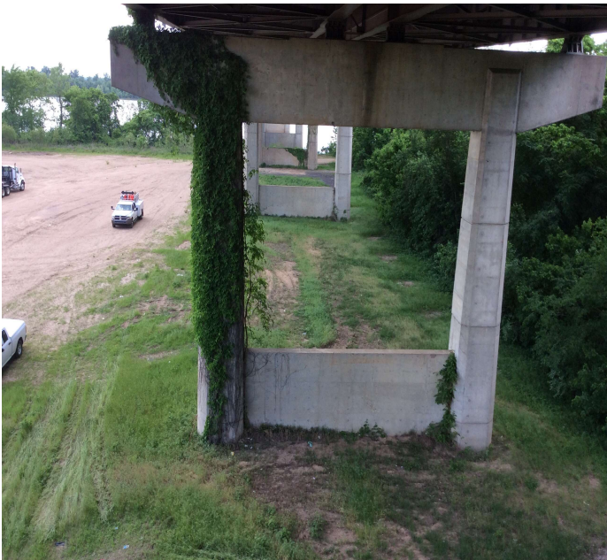
PHOTO 1 Description Ahead side pier 18 vines climbing up column onto the cap.
