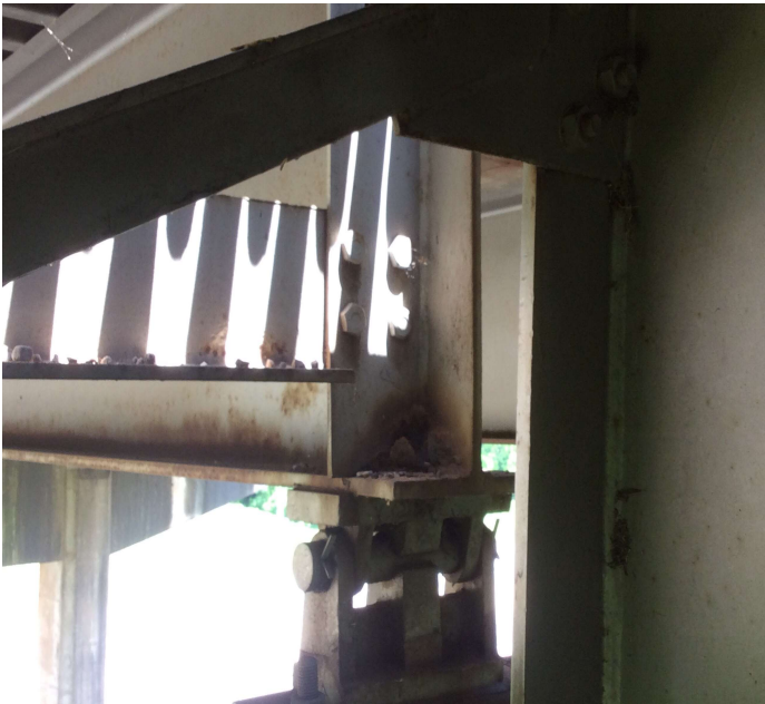
PHOTO 6 Description Pier 23: G5, Ahd: 3" hole corroded through bottom of girders vertical stiffener in bearing area.
