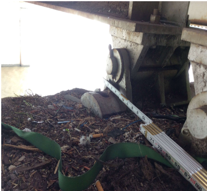
PHOTO 1 Description Pier 2 girder 5 both anchor bolts are missing at this bearing.
