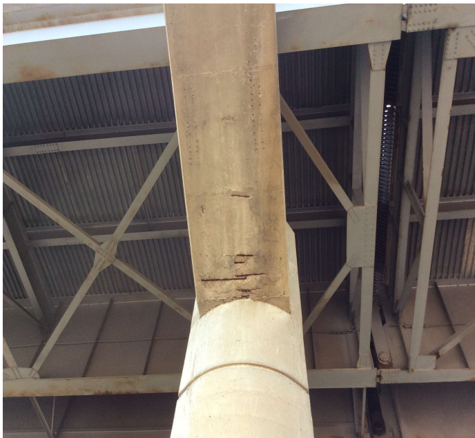
PHOTO 1 Description Bent 16 bottom cap right side Spalls with exposed rebar. This is the worst condition at this structure.
