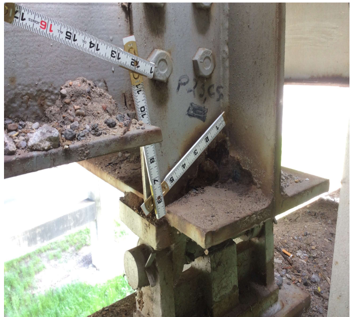
PHOTO 4 Description Pier 23 girder 5: a 2 3/4" by 1 1/2" hole at the bottom of the stiffener.
