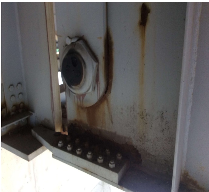
PHOTO 6 Description 13A Girder 3 1/8" section loss to web and 1/16" section loss to hanger bar. 1/4 pack rust
