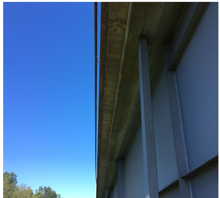
PHOTO 2 Description Span 17 loose utilities attachment.
