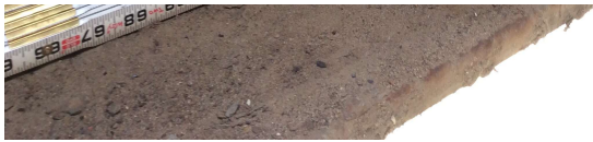
PHOTO 1 Description Left side of Girder 5 span 6 the last stiffener from the joint. Severe section loss to the lower section of the stiffener creating a 2" x 1 1/2" hole. Section loss also to the web and to the top of the bottom flange toward the joint at a length of 20". This is similar to Right side of girder 5 in the same span.
