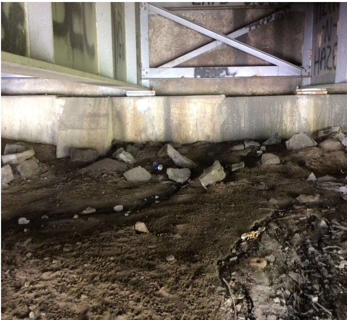
PHOTO 1 Description Abutment 1 Horizontal cracking in face.
