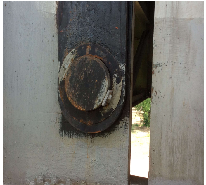
PHOTO 4 Description 17A girder 1 bottom pin. These pin and hanger assemblies have been repaired. This picture represents the repair work performed.
