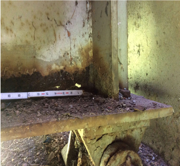
PHOTO 5 Description Pier 23 back Girder 4: Hole in Bottom of web 4 1/2" x 1".
