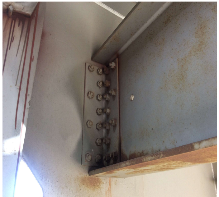
PHOTO 9 Description Pier 10 First Floor beam back on Girder 1 loose bolted connection.
