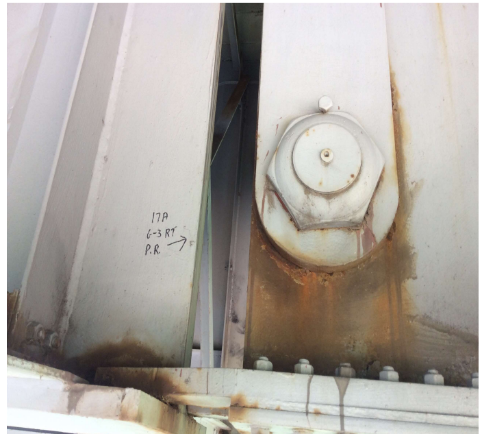
PHOTO 7 Description 17a Girder 3 pack rust with section loss in the hanger.
