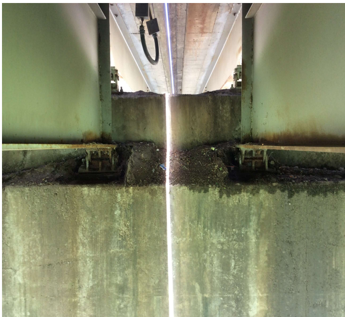
PHOTO 3 Description Debris has accumulated from the joint on to the backside of pier 23 between girders 4 and 5.
