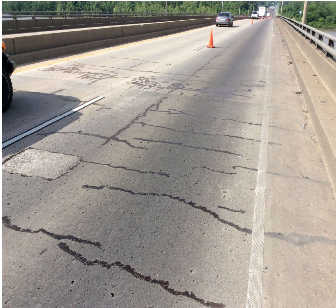
PHOTO 1 Description Southbound lanes. This is a common condition of the deck. Most of the transverse and longitudinal cracks have been sealed.
