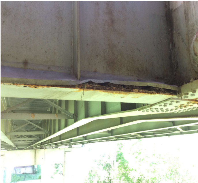
PHOTO 6 Description Joint 20A Protective cover failing active corrosion.
