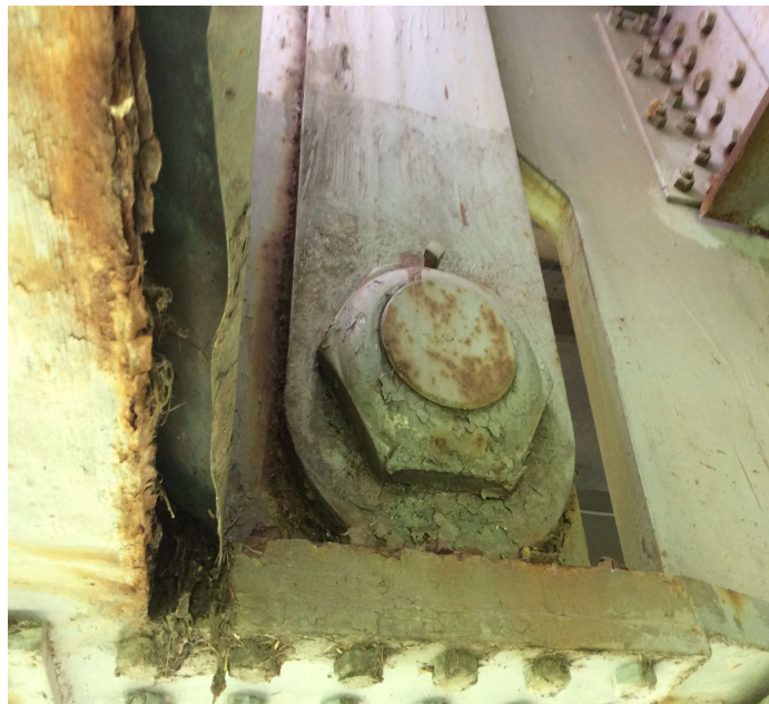
PHOTO 6 Description Joint 20a Girder 2 Pack rust in the hanger bars with section loss.
