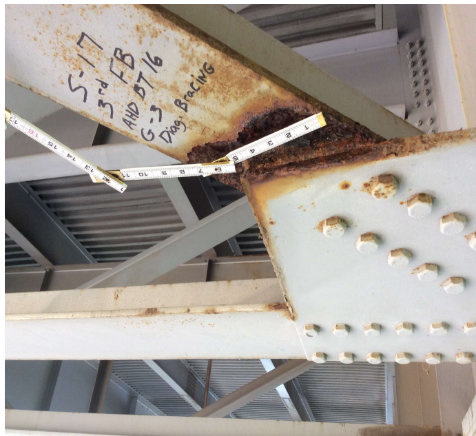
PHOTO 1 Description Span 17, girder 3 ,3rd floor beam at the diagonal bracing connection: Section loss up to 1/4 inch in a 7" x 3" area. Pack rust distorting gusset plate at this location.
