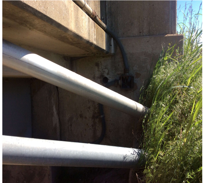
PHOTO 5 Description Abutment 2 right open junction box.
