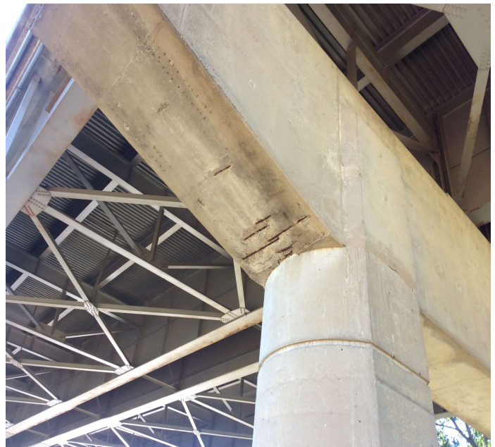
PHOTO 2 Description Bent 16 Right cap spalling with exposed reinforcing steel in under side of cap.
