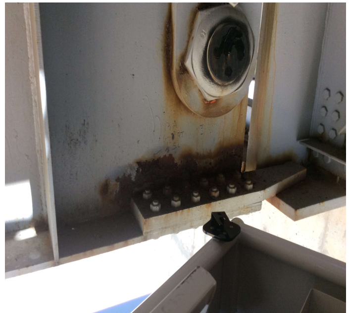
PHOTO 5 Description 13A Girder 2. 1/8 section loss to Girder 1/16 section loss to hanger bar.
