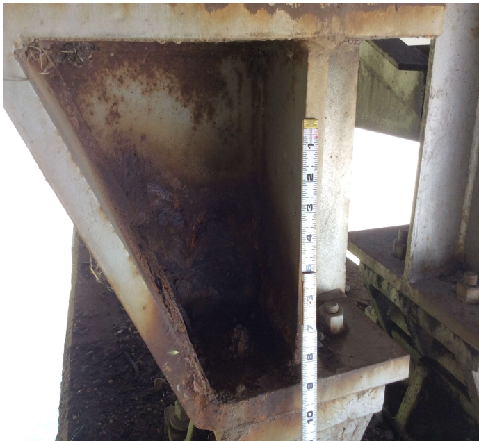
PHOTO 2 Description Span 2 girder 4 in the built up section at the end of the girder at pier 2. Dirt and debris from the joint is causing laminating rust at this location and also at girder 5.
