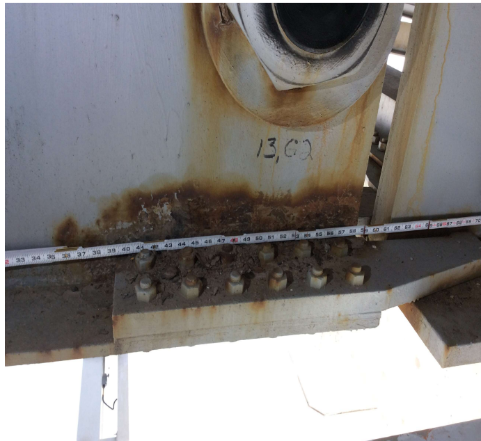
PHOTO 1 Description 13A, girder 2 above the wind lock: a 20" long by 4" high area of laminating rust. Typical condition to all wind locks.
