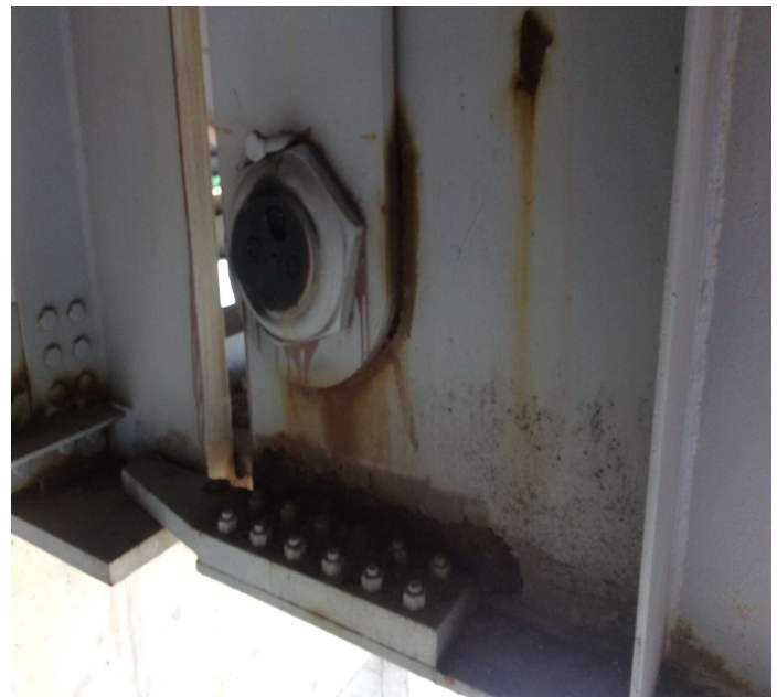
PHOTO 8 Description 13A Girder 3 1/8" section loss to web and 1/16" section loss to hanger bar. 1/4 pack rust
