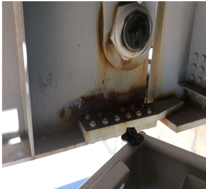
PHOTO 9 Description 13A Girder 2. 1/8 section loss to Girder 1/16 section loss to hanger bar.
