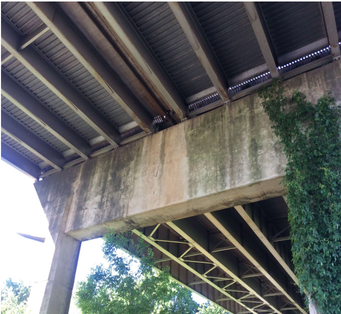
PHOTO 4 Description Pier 23 Delaminations in the face of cap.
