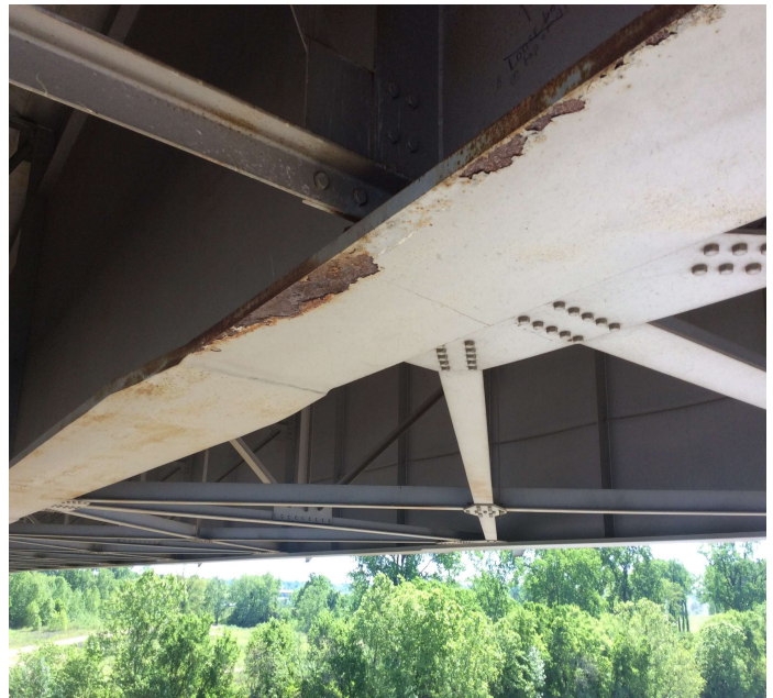
PHOTO 8 Description Span 15 Girder 3 at the third diaphragm connection.
