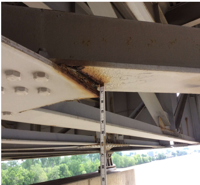
PHOTO 3 Description 13A Girder3 at the bracing and gusset plate connection has pack rust which is distorting the plate.
