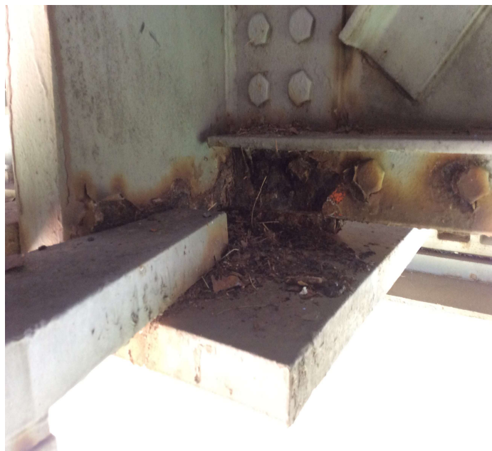
PHOTO 3 Description Joint 17A Girder 3 bolted connection reduced to nodes on two of four bolts.
