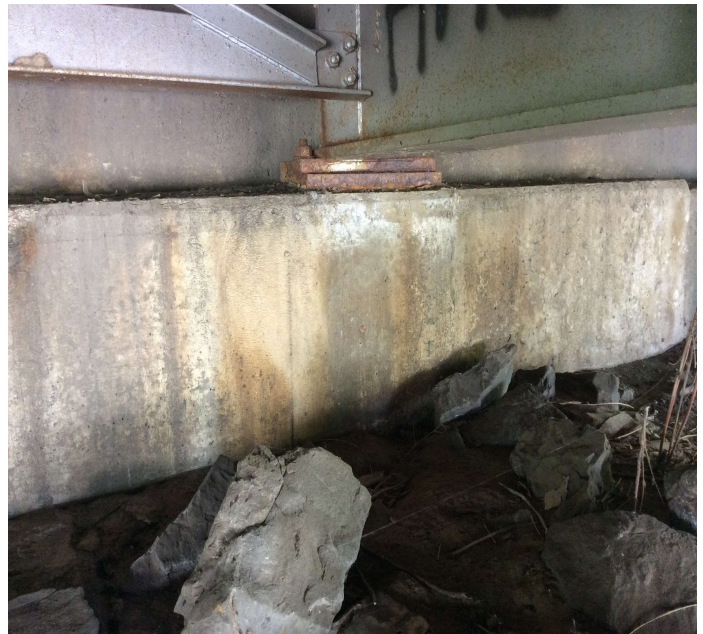
PHOTO 2 Description Abutment 1 girder 2: active corrosion and laminating rust to bearing, this is a typical condition of bearings at this abutment.
