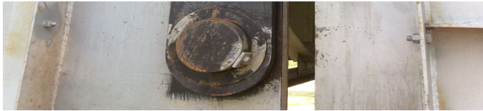
PHOTO 1 Description 17A girder 1, This pin and hanger assembly has been repaired. This picture represents the repair work performed.
