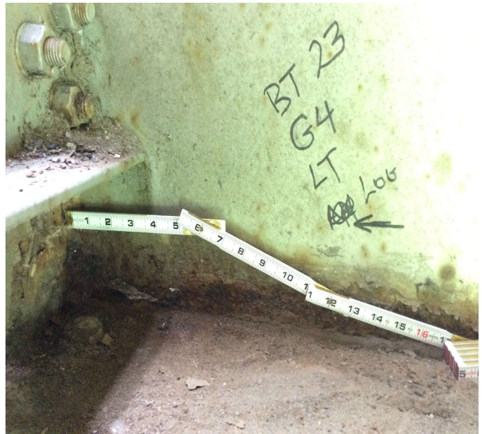
PHOTO 3 Description Bent 23, Girder 4: A 4"x1" hole in the web. Deep pitting to the lower web and flange. Girder 3 at this bent has deep pitting and section loss to its lower web and top of the bottom flange.
