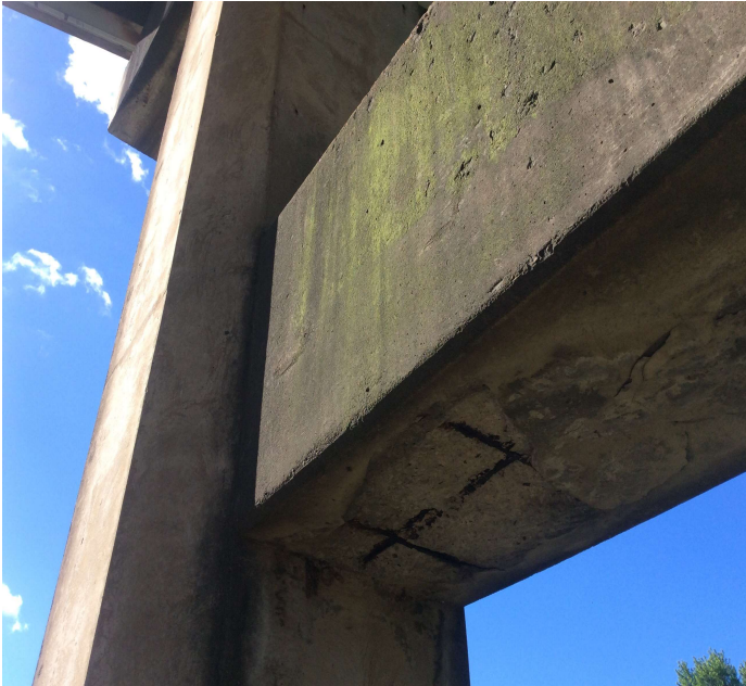
PHOTO 3 Description Pier 24 Spalling with exposed reinforcing steel on under side of cap.
