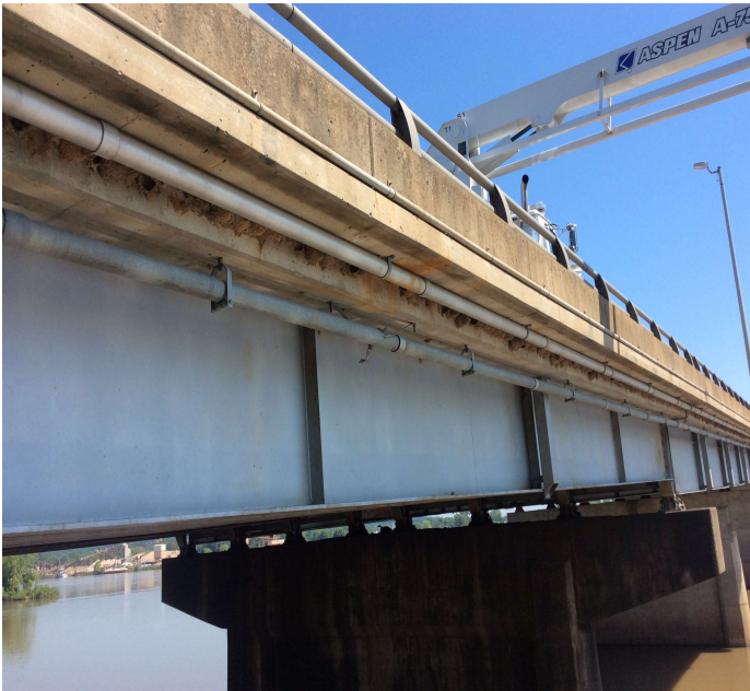
PHOTO 4 Description Missing brackets
