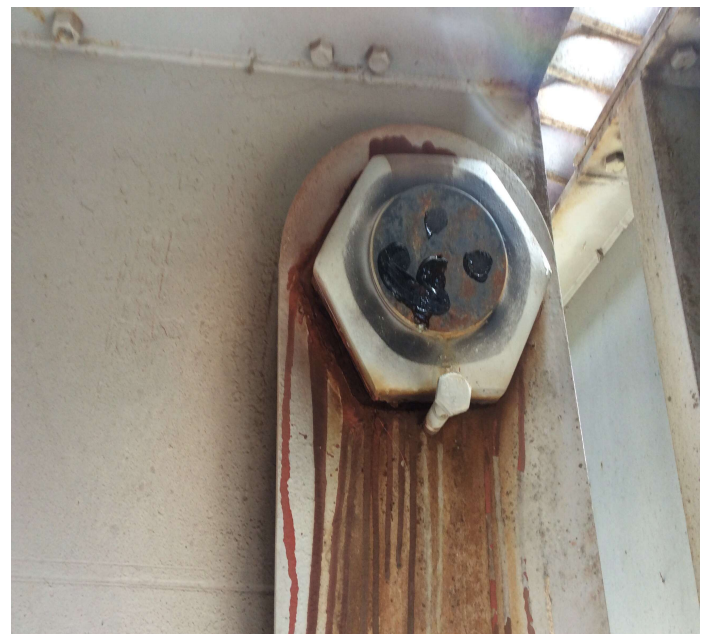
PHOTO 12 Description Joint 10A Girder 3. 3/16 section loss to the hanger bar.
