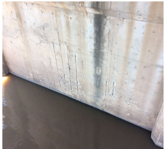
PHOTO 2 Description Pier wall: 1 spall with reinforcing steel exposed.
